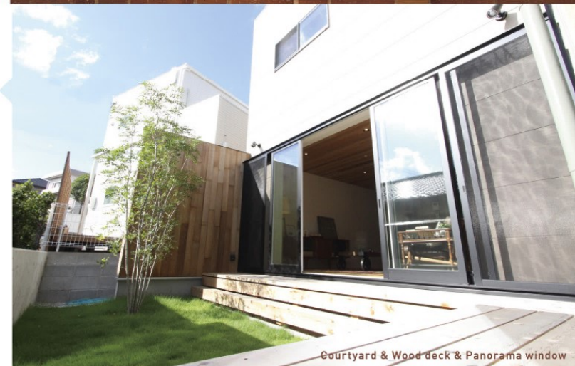
Courtyard & Wood deck & Panorama window
